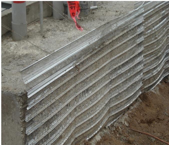
**STAY-FORM®** is a concrete forming system made specifically for constructing concrete encased duct banks. Designed with convenience in mind, the system eliminates the need for traditional concrete forms that can be quite the hassle to remove and clean.
